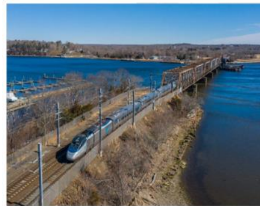
Susquehanna River Bridge Replacement
